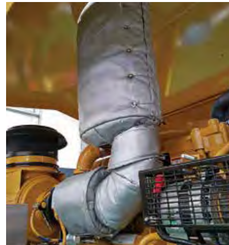
Thermal protection covers on exhaust, turbo and mufflers
